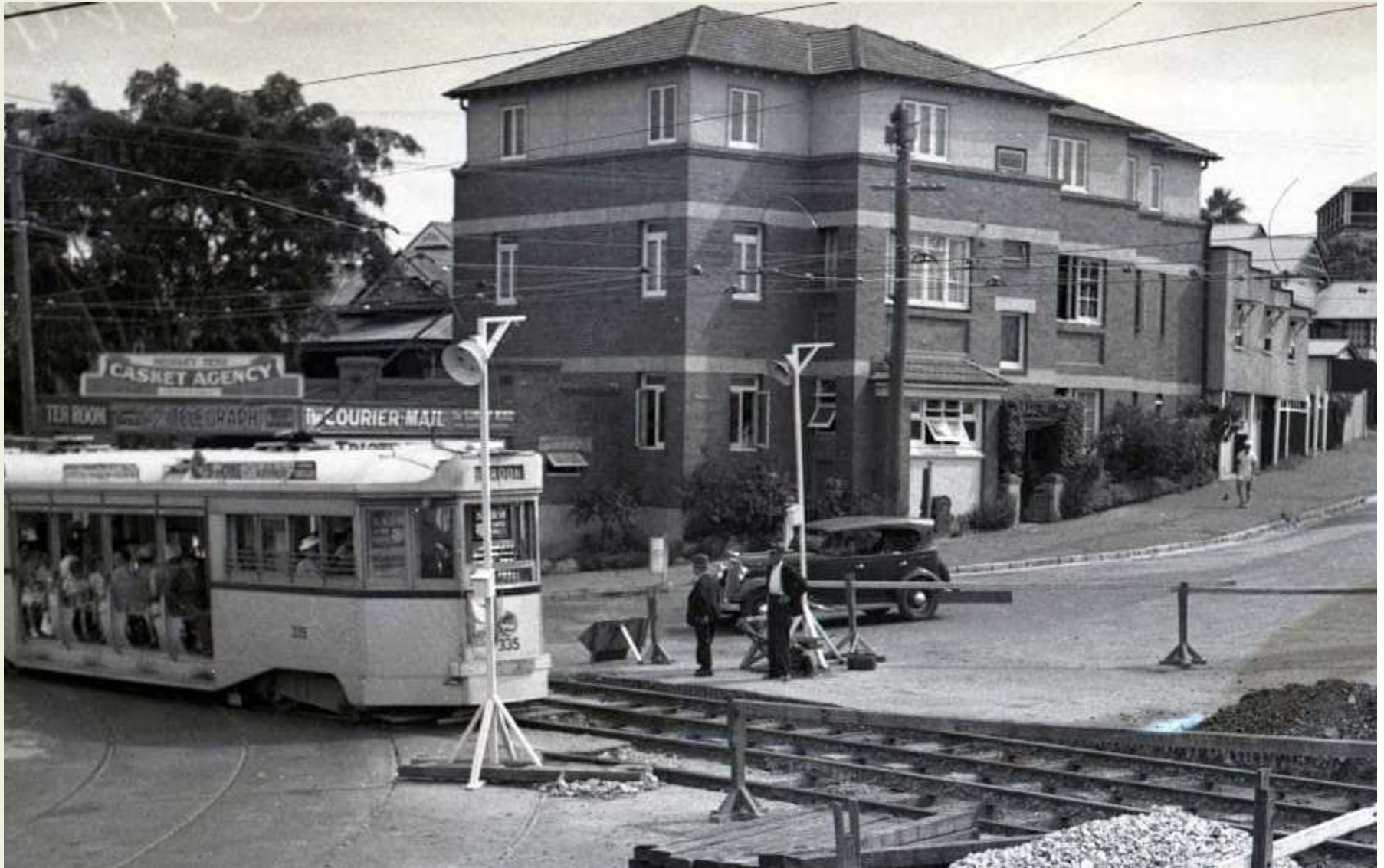
single tram crossing at Gregory Terrace Source. Courier Mail
